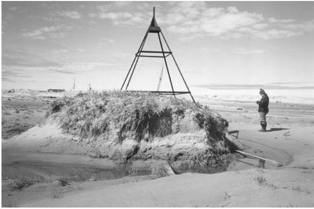
Fig. 7 During the period of exploitation, the surface of the barrier beach on Varandei Island sank 1–3 m due to deflation and thermoerosion
