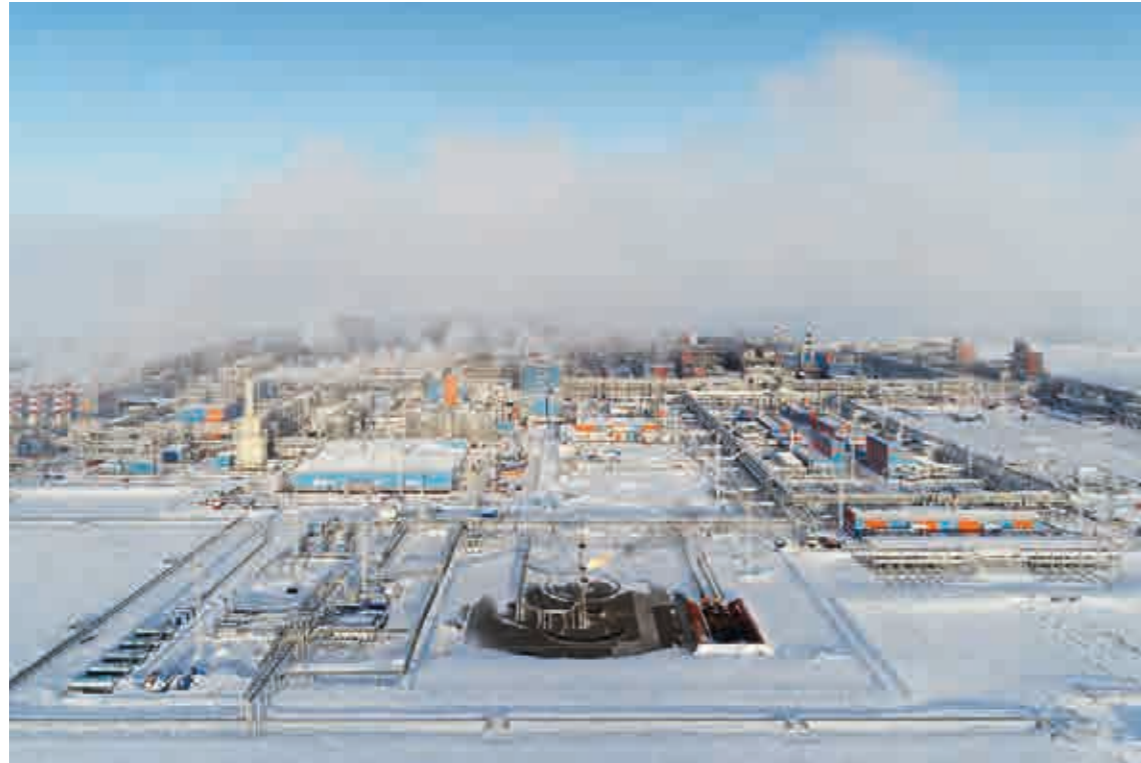
5.13 > The Russian company Novatek and its partners have built the Yamal LNG liquefied natural gas plant on the north-eastern shore of the Yamal Peninsula. In three production lines, natural gas is produced, liquefied and shipped to Europe and Asia via the port of Sabetta.
