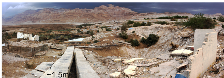
Figure 12. The impact of the sinkhole hazard near the shoreline. Photo taken by Djamil Al-Halbouni, modified after [70].
