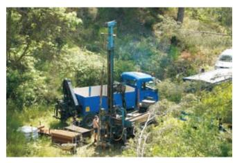
Figure 2. Drilling operations at section LB1 with a trailer-mounted rig.
