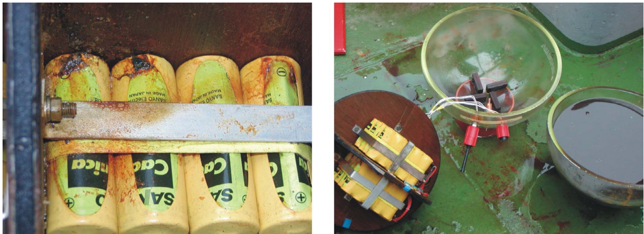
Fig. 5.9.2: Deformed and flooded Ni-Cd cells recovered during the first HDSD deployment.
