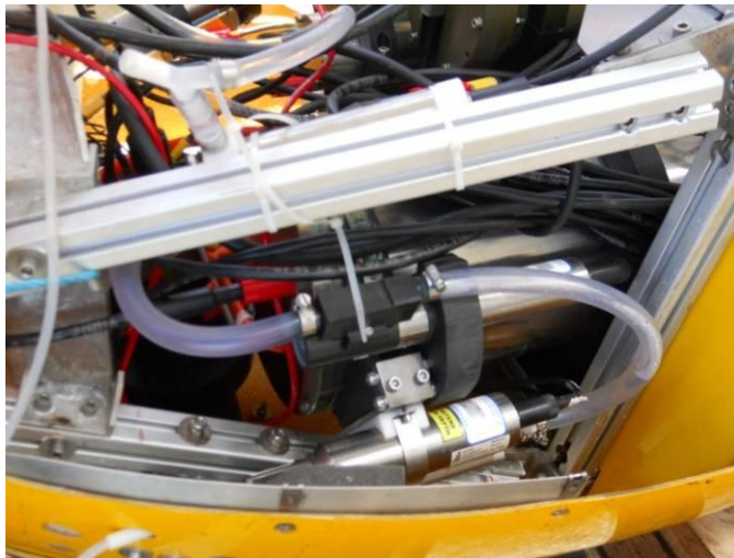
Photo 1. Port CT (mounted below the panel split line) and Oxygen sensor uppermost
