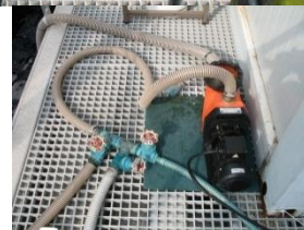
CO 2 neutral cooling with deep fjord water
