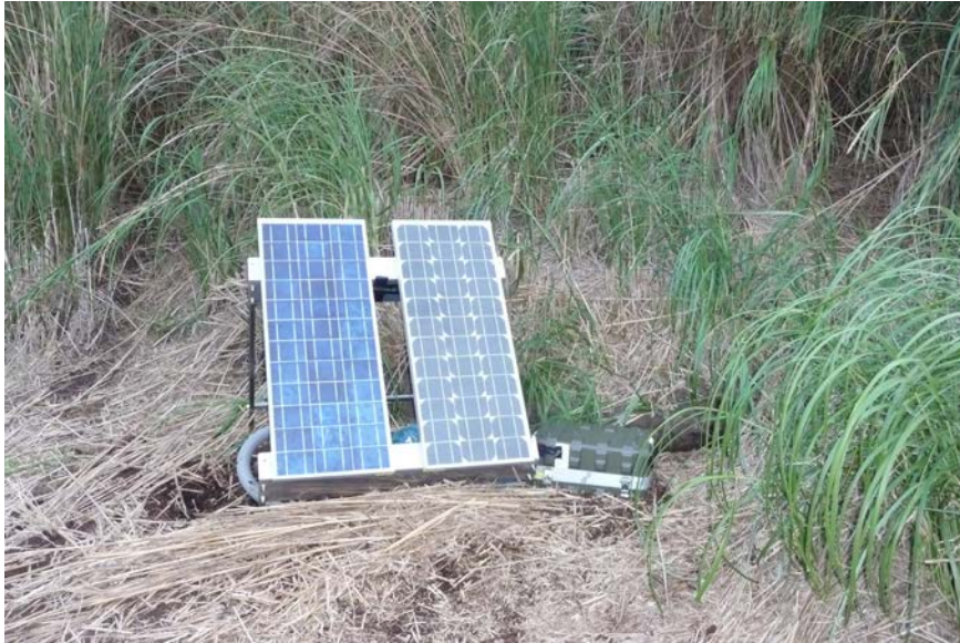
Fig. 5.3.4 Final setup of station NIG01. The seismometer is placed beneath the solar panels. This might be a potential problem during windy days.
