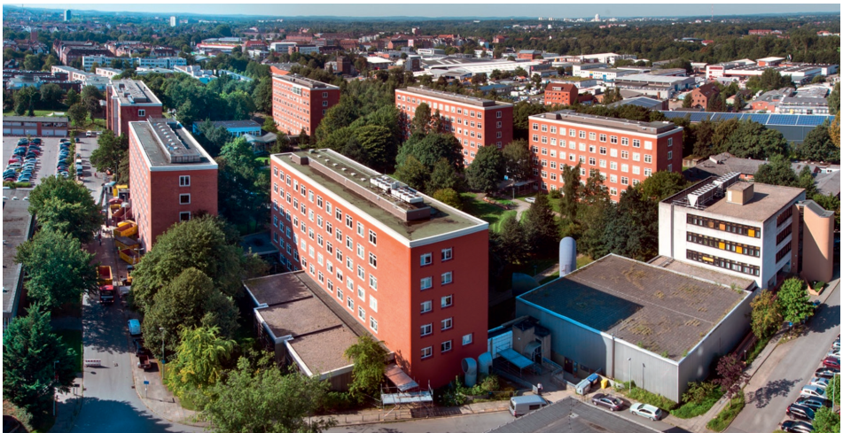
Fig. 3b. Picture of the “Angerbauten” in the Ludewig-Meyn-Strasse of the CAU campus which had been built in the mid-sixties, but which will be demolished in the near future because of constructional deficiencies. The new GPI (from 1967 onwards) as part of the “Angerbauten” is located on the far left corner of this group of buildings. The art of the building was modest at that time with the result that a decision has been reached in 2015 to demolish it and to plan for a new building, also as part of the CAU campus, but at some distance to this location. (Photo by permission of Volker Rebehn, Kiel)
