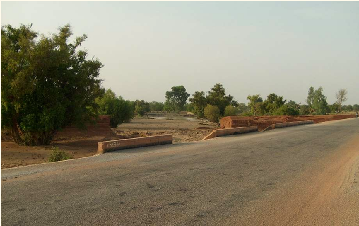
Figure 15. The newly paved road RN22.
