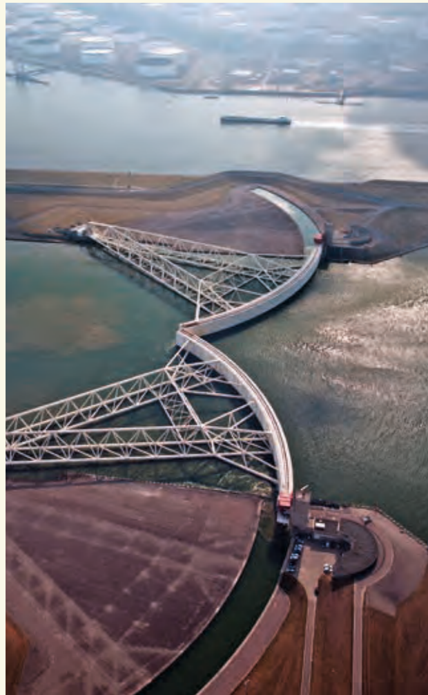
4.18 > The arc-shaped gates of the Maeslant Barrier close when the Rotterdam metropolitan area is threatened by a storm surge. It protects the city and the port from high water levels.
