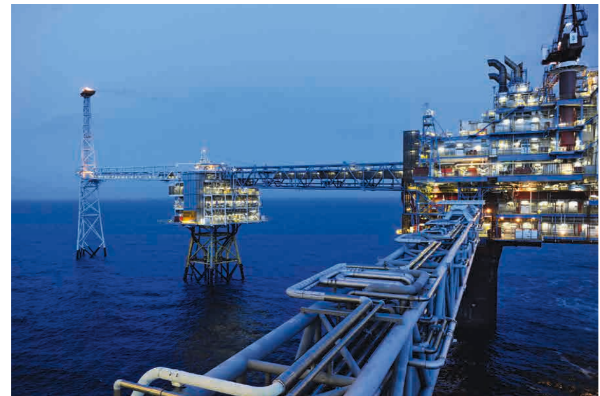
5.24 > In the Sleipner gas field in the North Sea, carbon dioxide that rises to the sea surface during the production of natural gas is captured directly on site, liquified, and then injected at a depth of 880 to 1100 metres back into the seabed.
