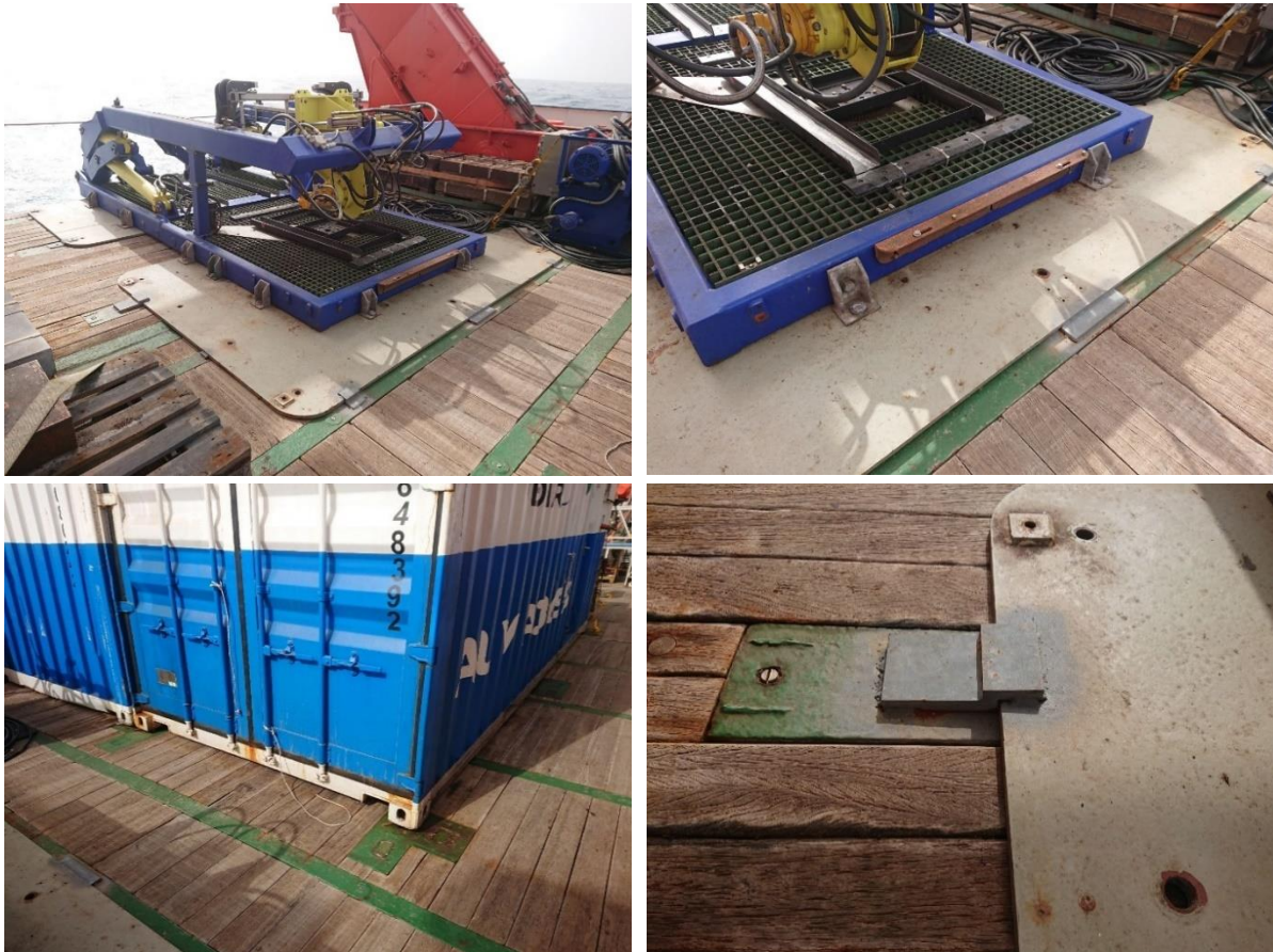
Fig. 12.4 Top left: Launch and recovery system (LARS) on aft deck of RV METEOR. Top right: Mounting of the LARS on deck via steel plates. Bottom left: Container for AUV operation. Bottom right: Steel plates are temporary welded to the aft deck via Z-profiles.
